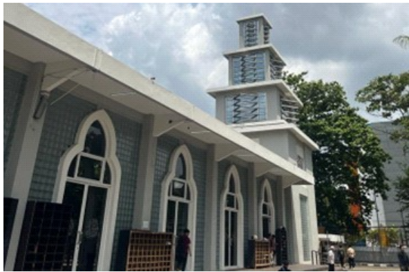
Figure 2. Front View of UIN Sunan Kalijaga Campus Mosque.
